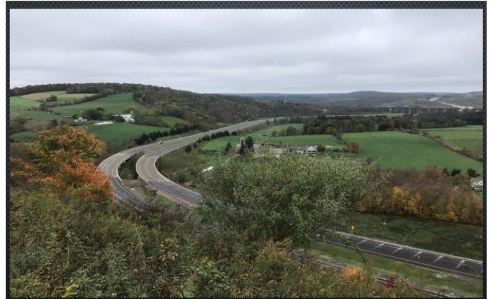
PENNDOT DISTRICT 9-0, GULISEK CONSTRUCTION & QUAKER SALES CORP
