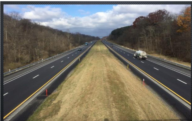
PENNDOT DISTRICT 12-0, LINDY PAVING INC.
