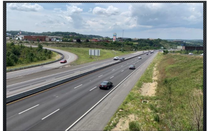
PENNDOT DISTRICT 11-0, LINDY PAVING, INC.
