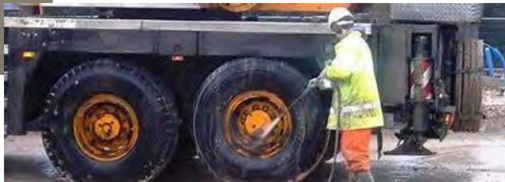
Wheel Washing to Remove Sediment
