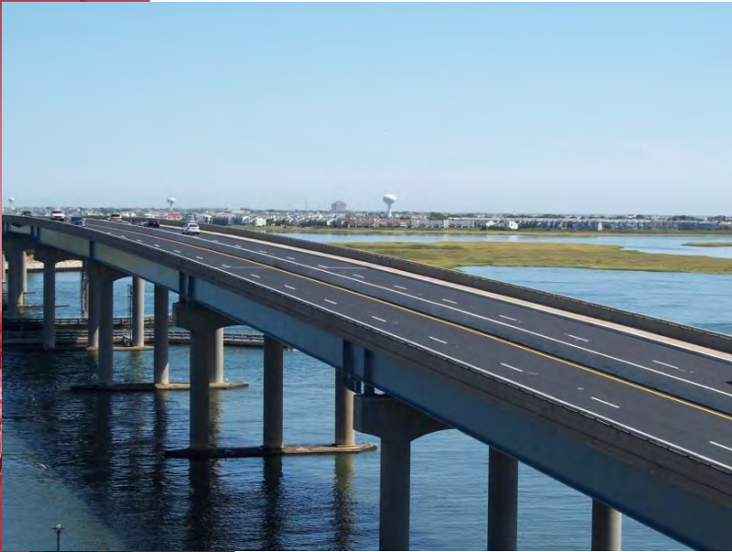
NJ Route 87 Absecon Inlet Bridge
