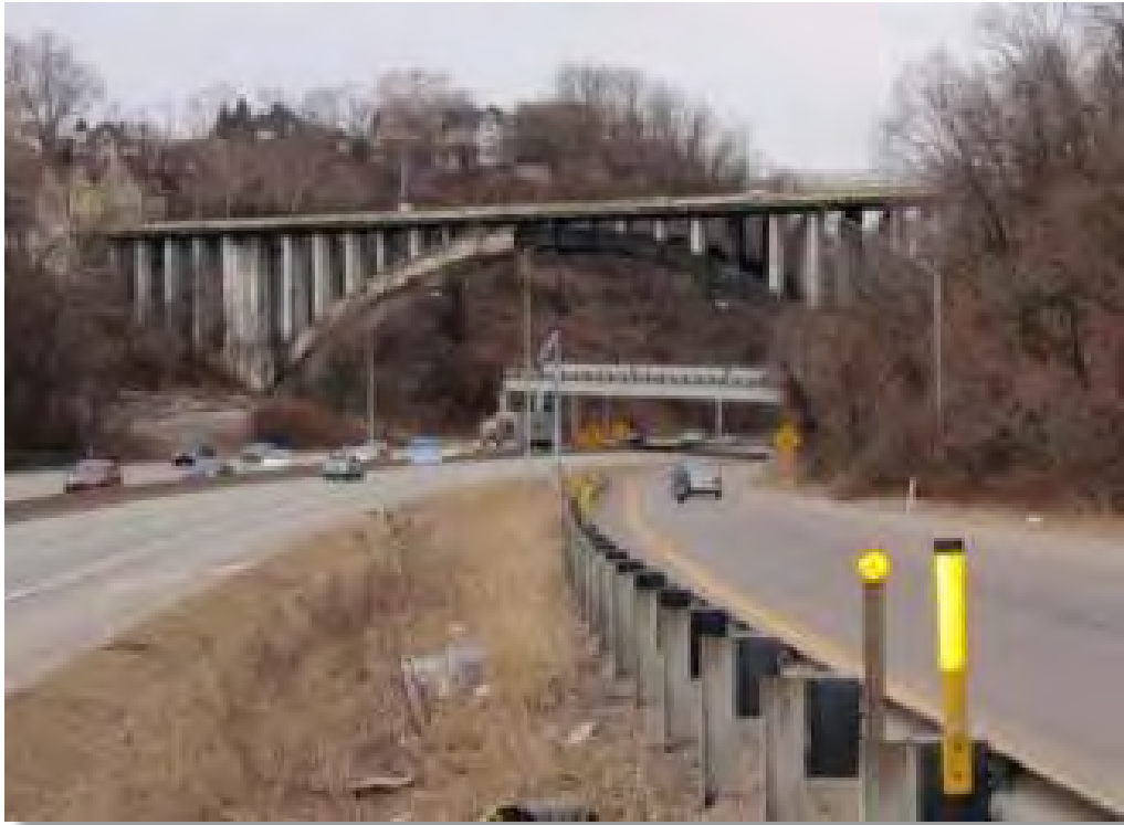
Greenfield Ave. Bridge City of Pittsburgh
